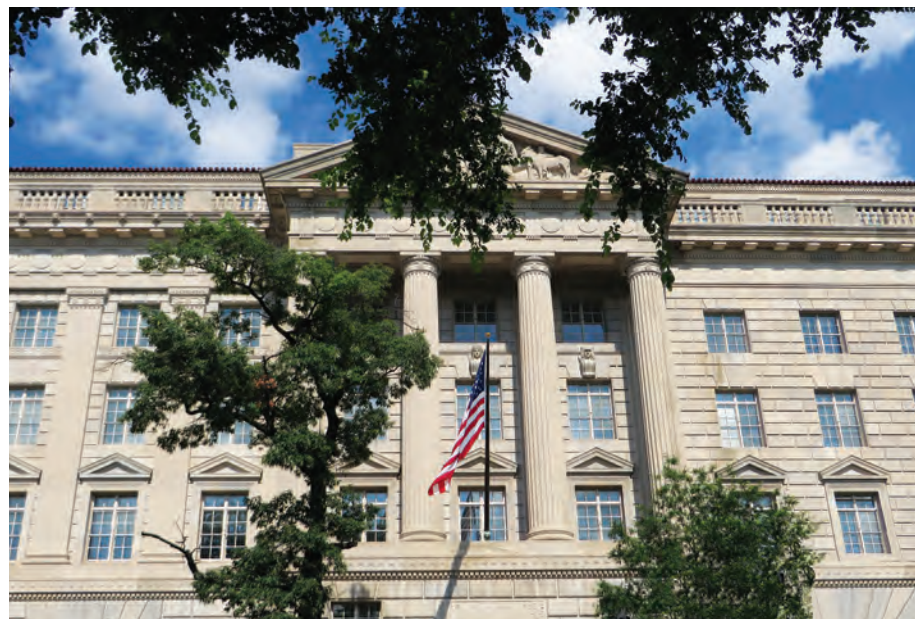
U.S. Department of Commerce Building — Washington, D.C. • Interior Blast Guard Windows
