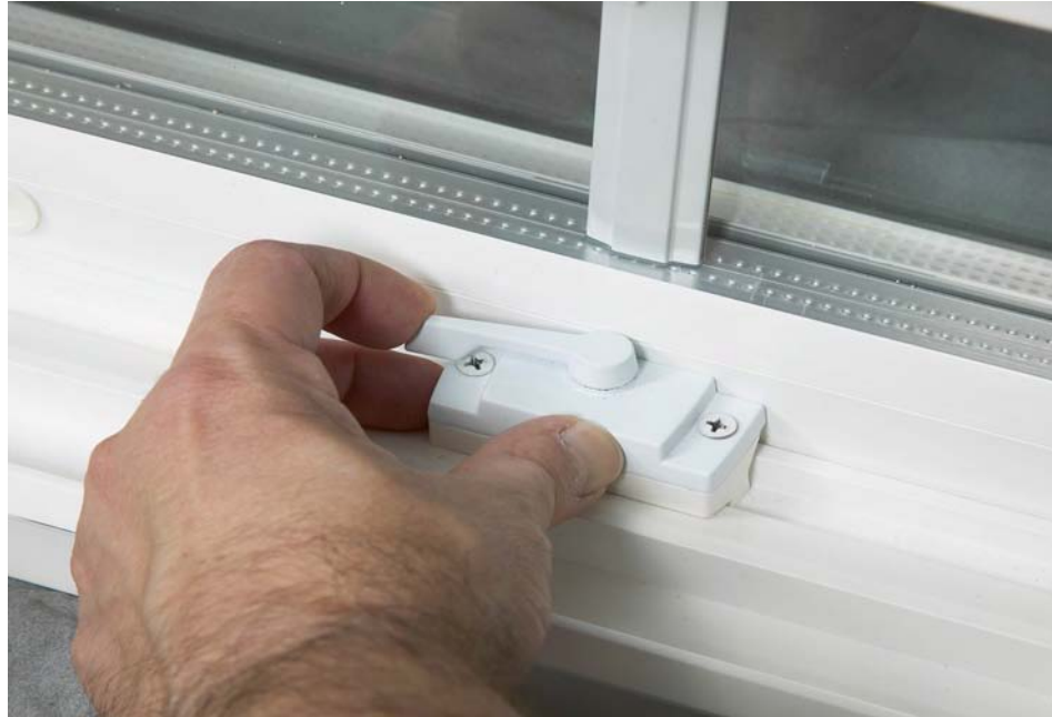
Photo 4 Unlock exterior bottom sash.
