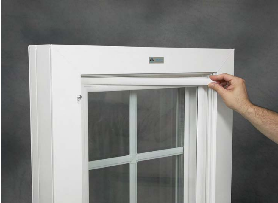
Photo 32 Top glazing bead removal.
