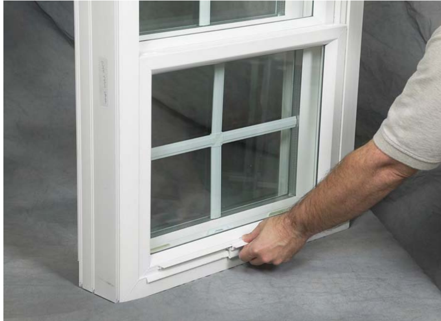
Photo 2 Unlock interior bottom sash.
