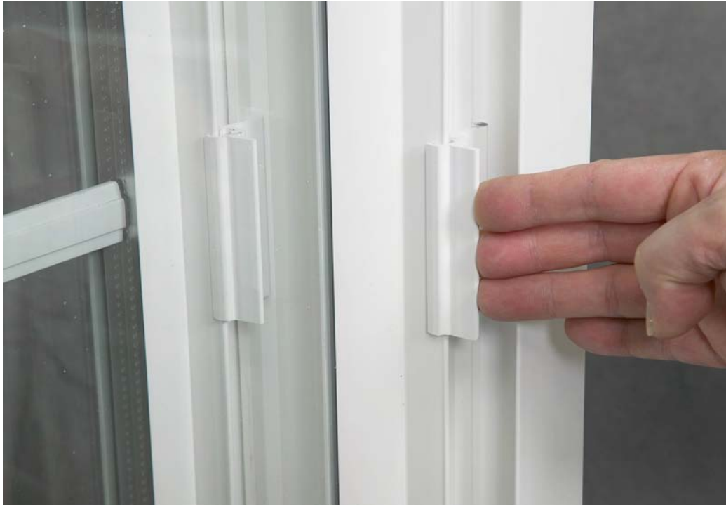
Photo 20 Release sash lock.
