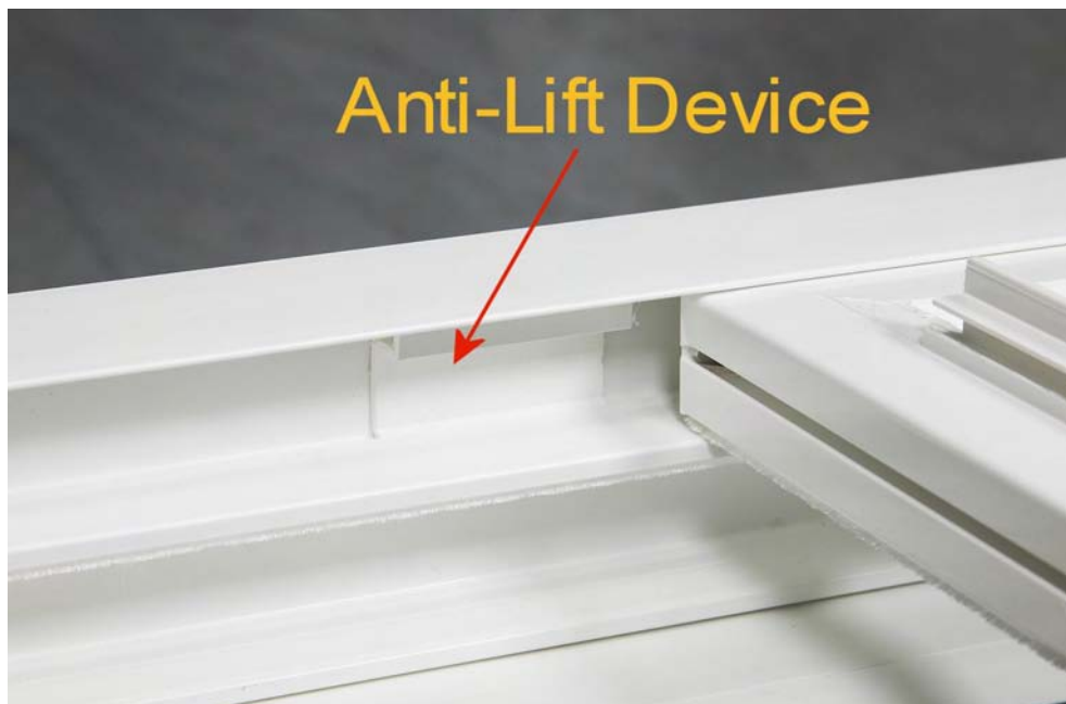
Photo 21 Open sash past anti-lift device.
